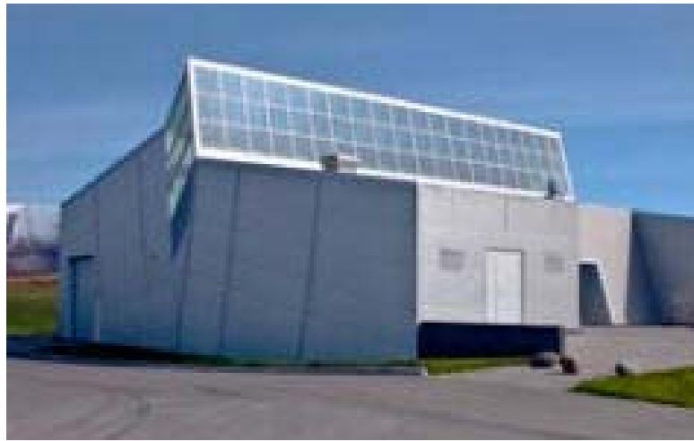
Figure 2.7 Kalina cycle geothermal power plant in Iceland [26]
